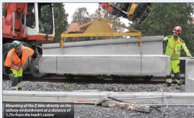
*Mounting of the Z-bloc directly on the railway embankment at a distance of 1.7m from the track's centre*
